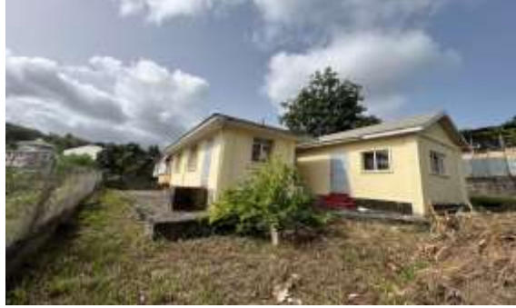
Side and rear view
